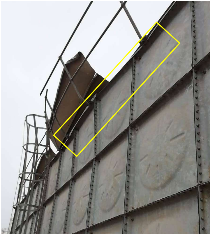
Figure 4 Damaged Side Panels Located on the Eastern Wall of the FWT
